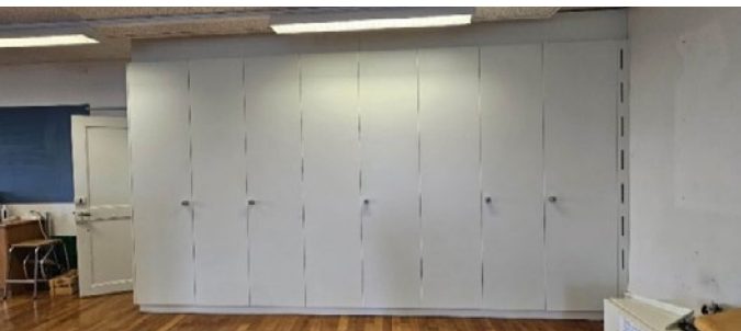
Installation de placards
